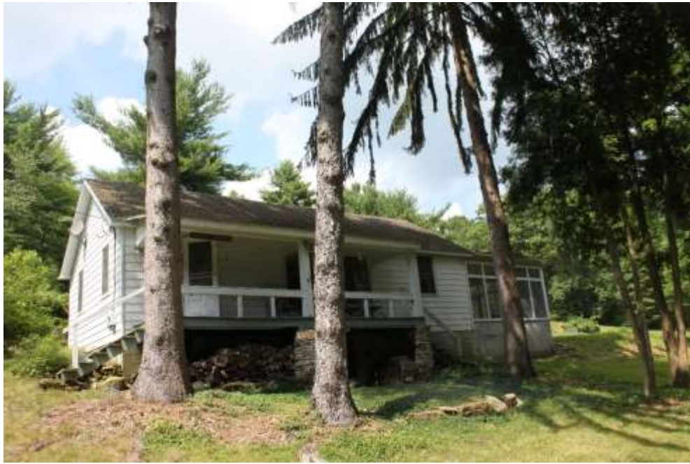
One of the three remaining structures of the camp is the Officers' Quarters shown.
