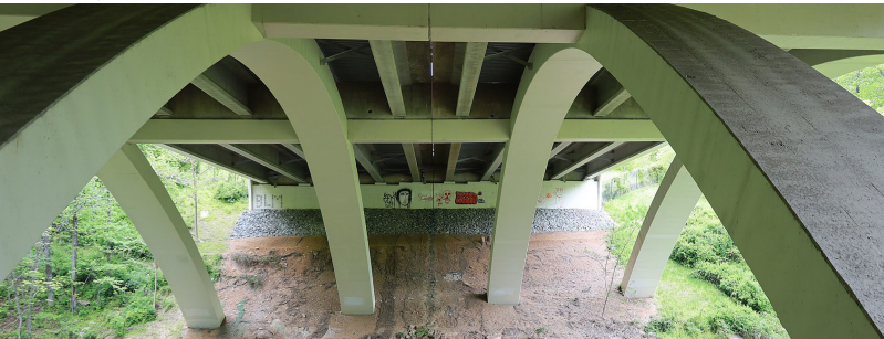
Image: MD 200 crossing Rock Creek, wide arch facilitates wildlife crossing credit: wikiwand.com
