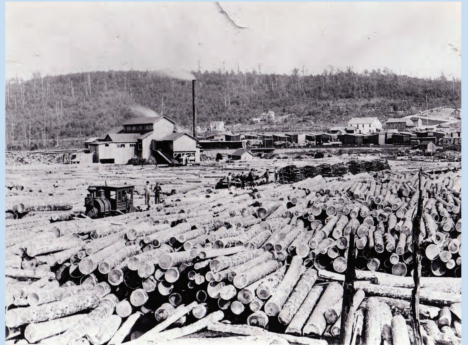
During the logging railroad boom in Centre County, trees were cut, stripped of their branches, and piled along a railroad line where they were picked up and transported elsewhere. Collections of the Centre County Historical Society.
