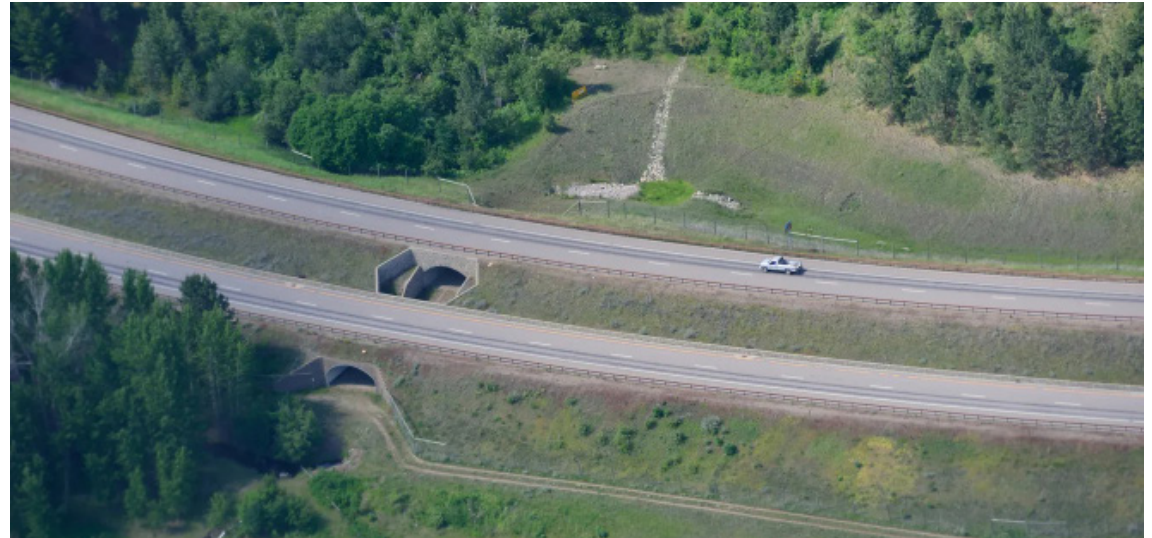
Figure 1.11 - US 93 - Flathead Reservation - Montana
