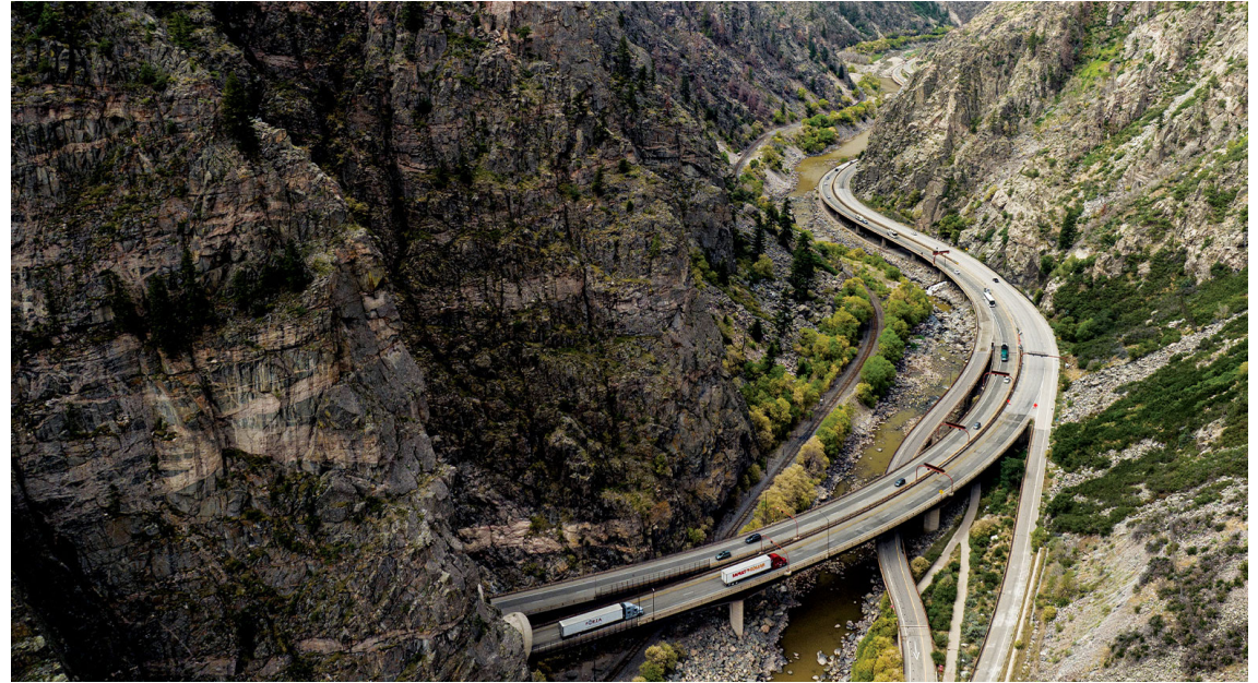
Figure 1.02 - I 70 - Glenwood Canyon, Colorado
