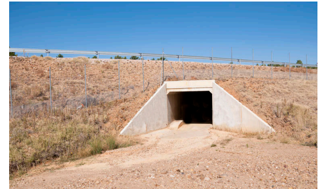
Soria, Spain A-15 Motorway
