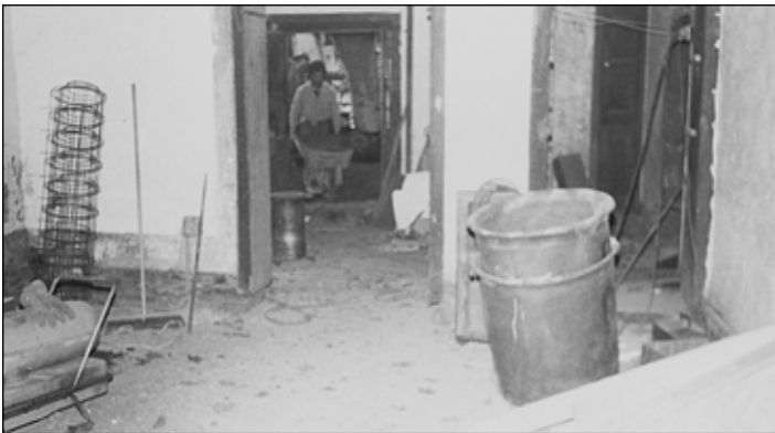
Hearth Room looking towards the Museum Store, c. 1984.
