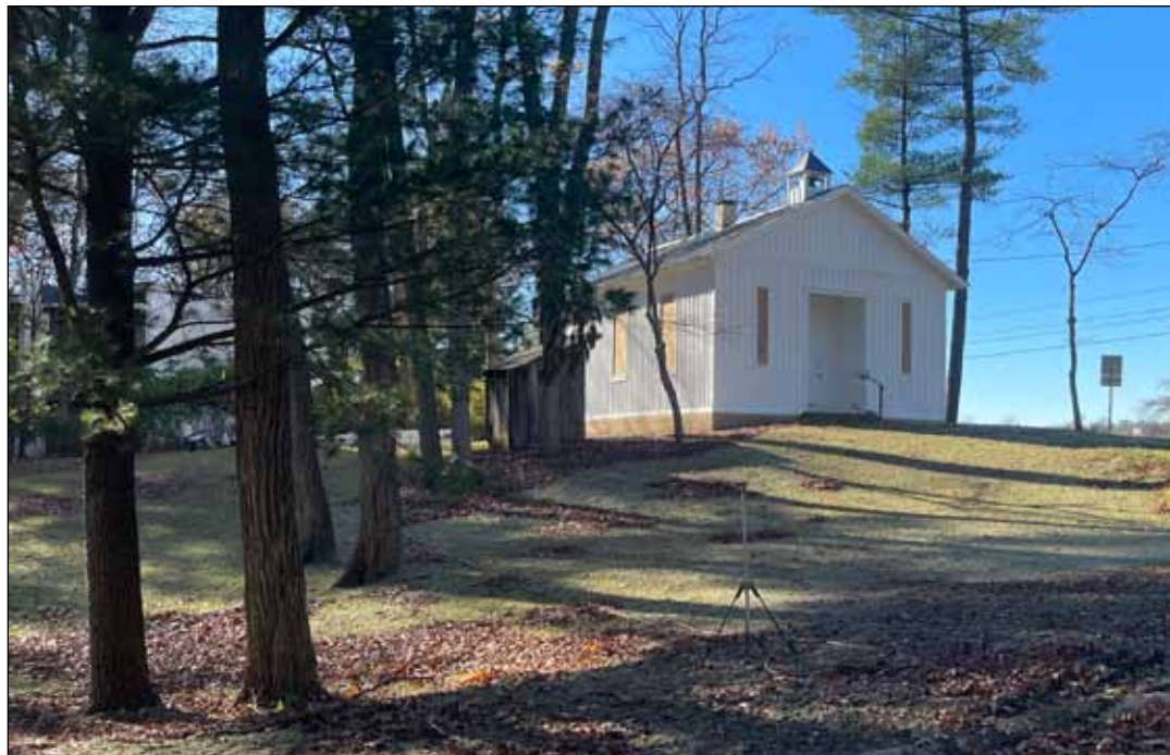
Boogersburg School landscape and building work as of November 1.
