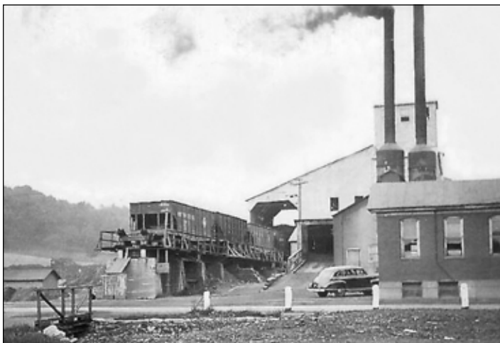
The Snow Shoe brickyard at Clarence about 1949, showing the trestle where coal was unloaded to fire the kilns. Photo provided by author.
