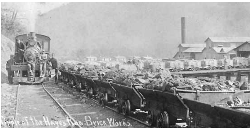
A narrow gauge or "dinkey" railroad brought raw clay from the mine to the Hayes Run brickyard at Orviston. Photo provided by Jim Davy.
