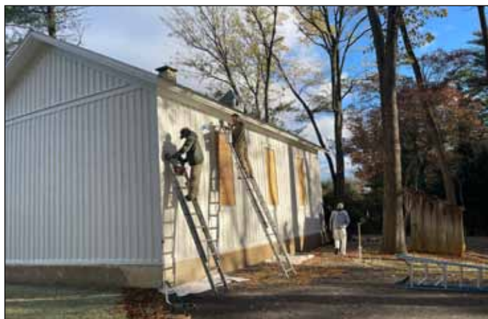
Exterior painting by Home Wrights Construction.
