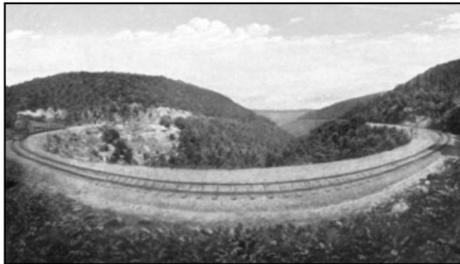
A postcard view of the Big Fill on the PRR's Clearfield Branch. The massive earthen fill enabled trains to cross the valley Pleasant Run on the Allegheny Front. Provided by author.
