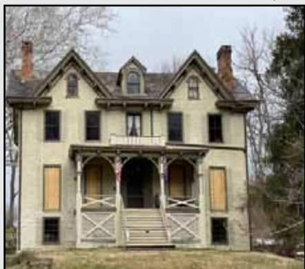
Notice the absence of shutters and windows - soon to change!
