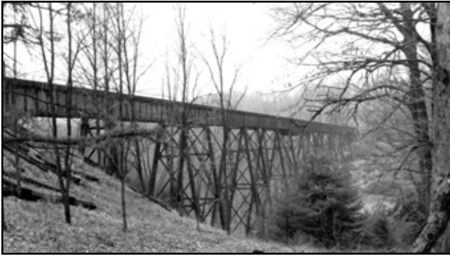
The Beech Creek Railroad's viaduct across the Moshannon Creek. This view looks toward the Centre County side. Provided by author.
