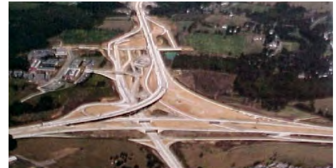
Image: [2002] Interstate 99 & U.S. 322 Interchange (PennDOT)
