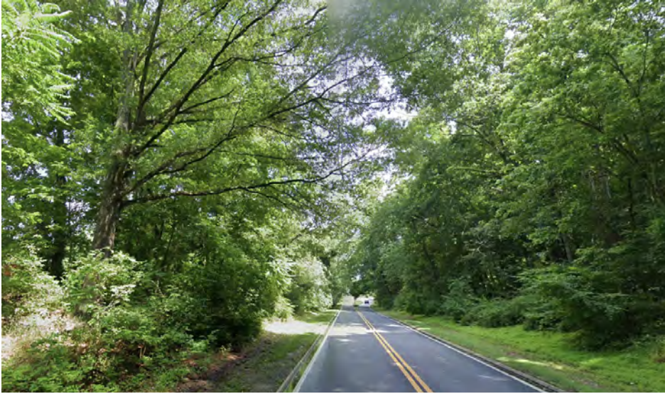
Figure 2.0 - Shows two-lane segment, Clara Barton Parkway.
