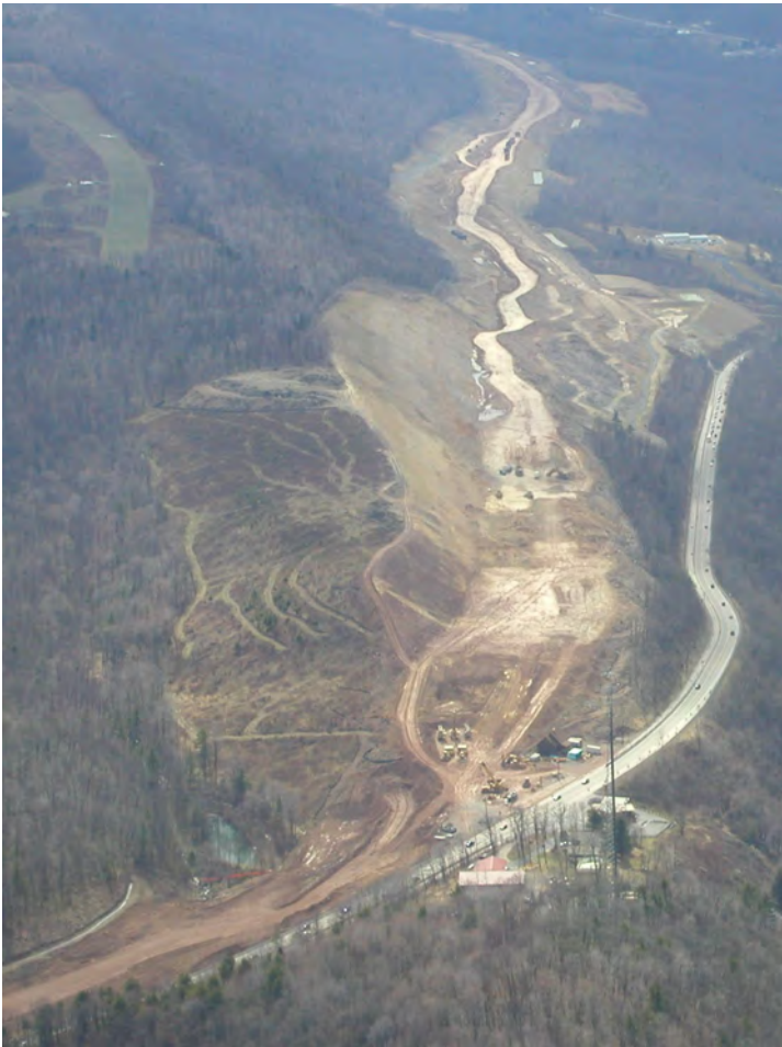
Image: [2002] Bald Eagle Mountain, Interstate 99
