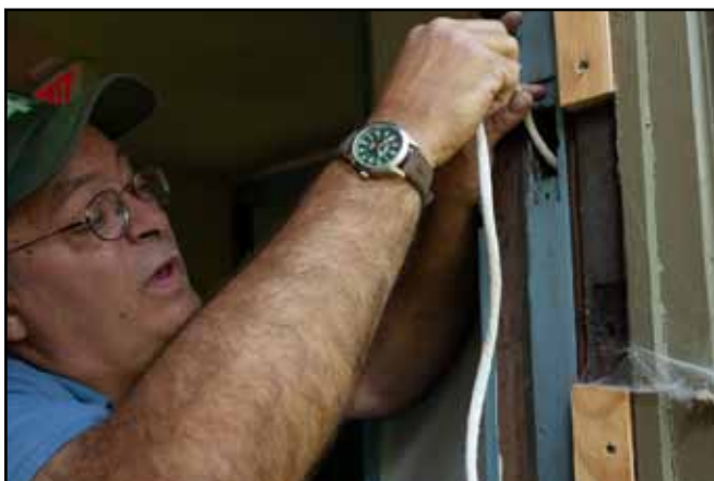
Replacing a cord pulley
