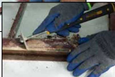
Paint removal after steaming
