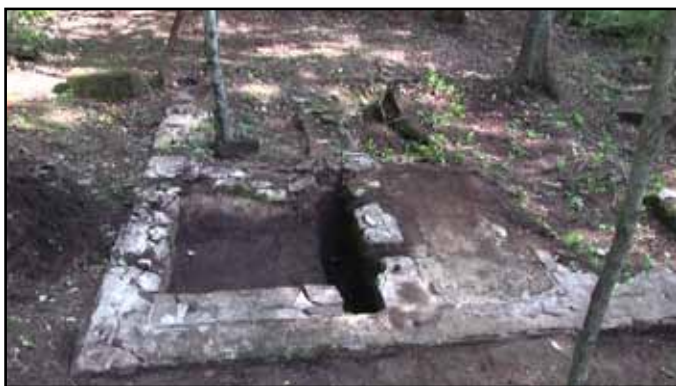
Wheel pit for one of the cable drums to pull ore cars up the incline three stories up and into the ore washer. Site work completed with Special Use Permit.
