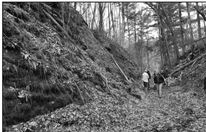
Several deep cuts had to be made in the landscape to keep the railroad bed level.
