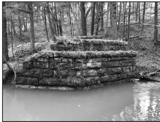
Railroad bridge abutment showing the meticulous stone work.
