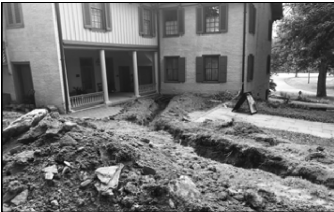
Top: Brick "patio" along the porch was removed before the trench was dug. Bottom: View of trench to the connection point at the rear of the Mansion.
