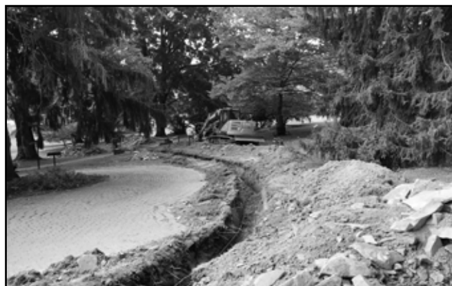
Top: The waterline trench is dug by Glenn O. Hawbaker from the Dogwood bed across the walkway. Bottom: The trench as it follows the curve of the driveway. Notice the limestone that was removed.
