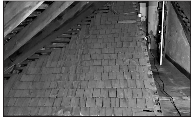
Below: Original 1830s shingles on the Mansion roof enclosed in the attic with the addition of the ell in 1846.
