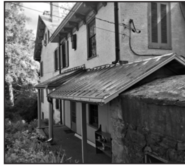
Clockwise from upper left: Balconied porch restoration with copper roof; view of the historic Sycamore from the balconied porch; front balcony and roof restoration; back porch with new copper standing seam roof and gutter system.
