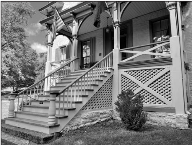
Front porch stairs of the Centre Furnace Mansion
