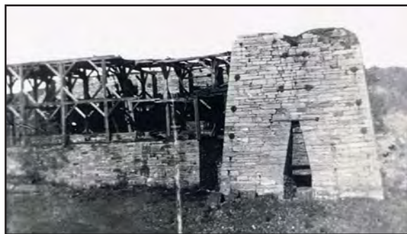
The second furnace at Pennsylvania Furnace. The structure to the left of the furnace contained all the machinery for steam power and hot blast operation. Circa 1930's.
